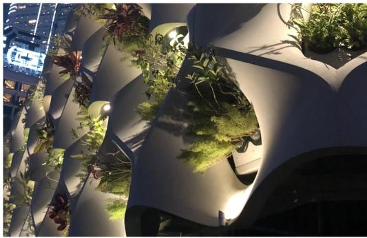
All light sources used in the Garden are LED, mounted with weatherproof, marine resistant enclosures. Balanced lighting scenes can be adjusted using a fully automated lighting management system.
